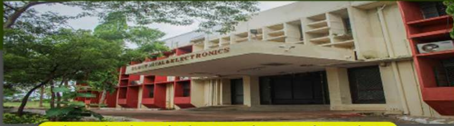
Electrical and Electronics Engineering
